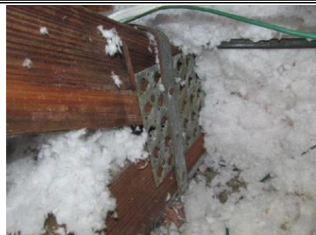
ROOF TO WALL ATTACHMENT (BACK)
