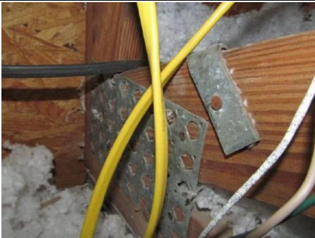
ROOF TO WALL ATTACHMENT (FACE)
