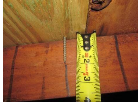
ROOF DECK ATTACHMENT (NAIL SIZE)
